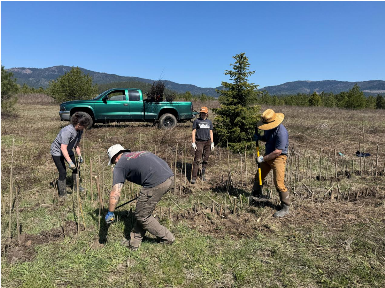
Photo 5: Dormant willows planted on WF Lake Creek, April 2025.
