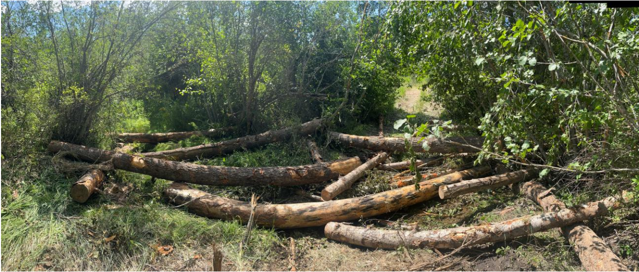
Photo 4: Floodplain/Channel wood additions in Bozard Creek.
